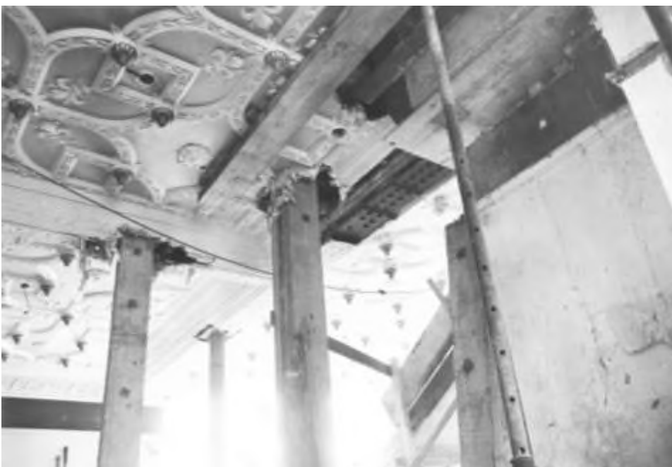
Kingerlee inserted wooden uprights to hold up the floor above whilst remodelling of the ground floor banking hall went on. The damage thus caused to the plaster ceiling was later repaired by the Herbert brothers. It's likely however, that the colours of the ceiling were lost at that point, and that it was painted all white, as it is today. Image (April 1978) courtesy of the Oxfordshire History Centre, Oxfordshire County Council, ref: POX0205301.
